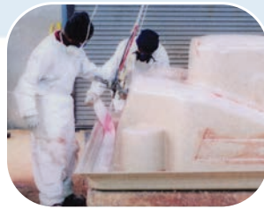
Fiberglass matting adds structural integrity in critical areas.
